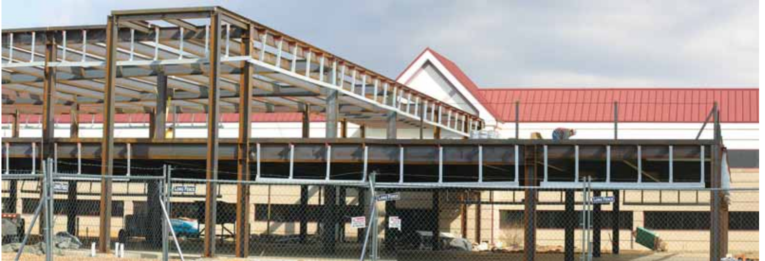
Above - Steel structure is being erected on the portion of the new medical center that will connect to the existing Robinwood Medical Center.
